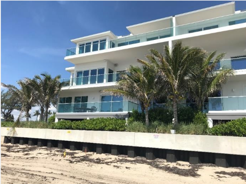
Areas with Poor Engineering
